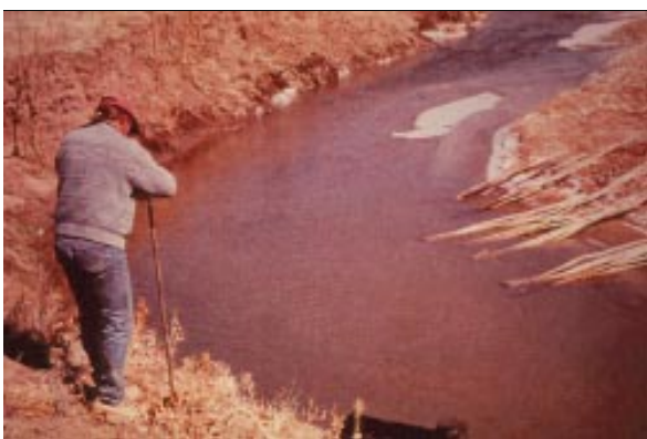
Figure 3. Cottonwood poles can stabilize stream
