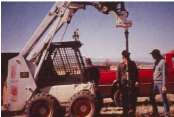
Figure 2. An auger creates a hole for a cottonwood pole.
