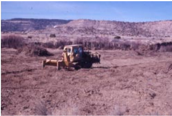
Figure 1. Vegetation can be removed with a rootrake.
